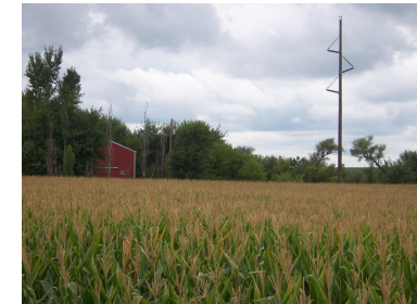
Above Ground Transmission Lines
