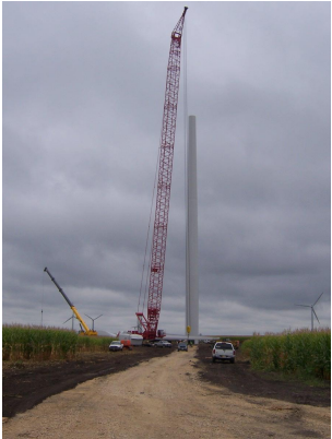
Tower and Access Road
